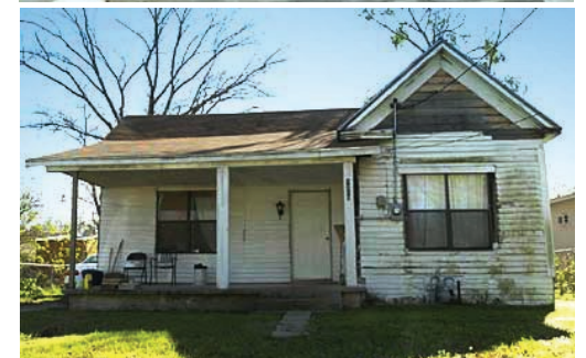
Top: the house after the fire. Bottom: the house as it was recently rebuilt.
